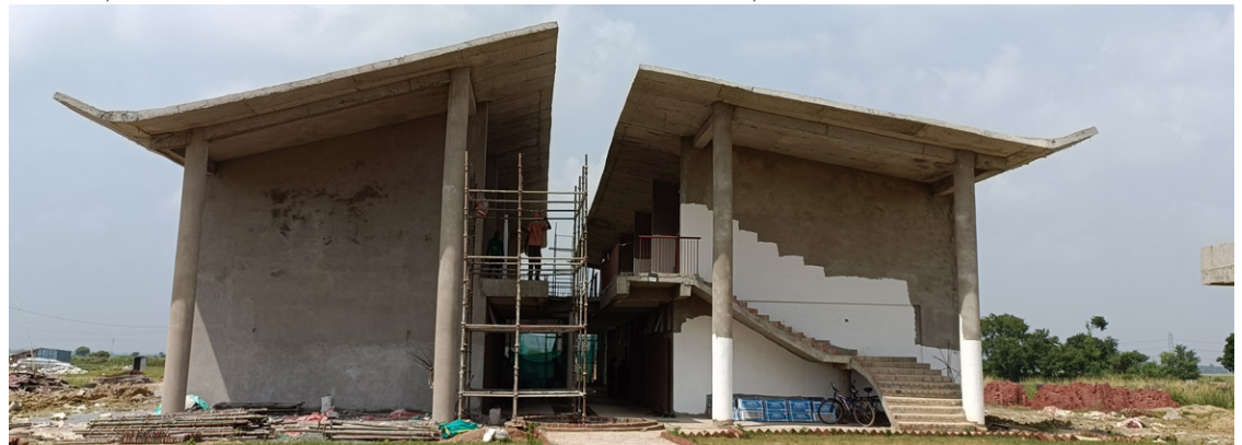
Phase 1, Junior Academic Block Under Construction- September 9, 2022
