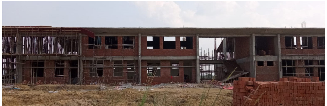
Phase 1, Junior Academic Block Under Construction- June 24, 2022
