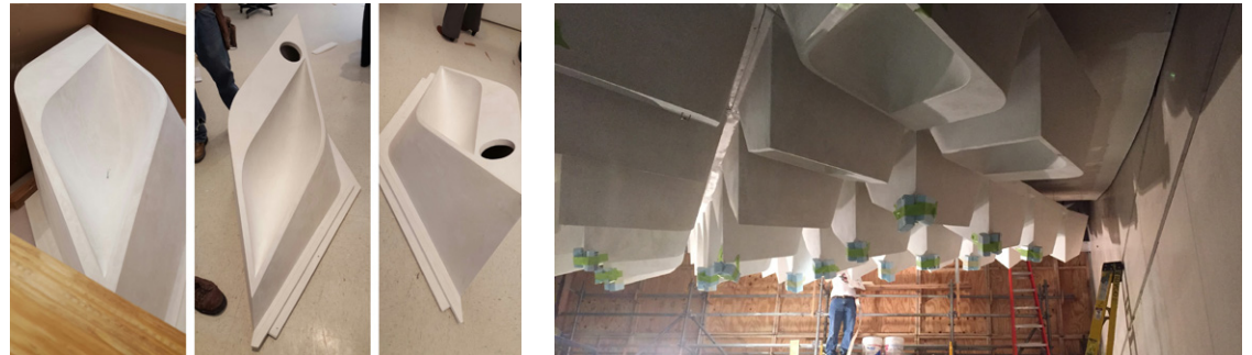
GFRG panels being installed on site
