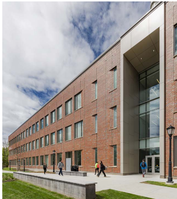
East brick façade is a new variation on the campus' masonry buildings
