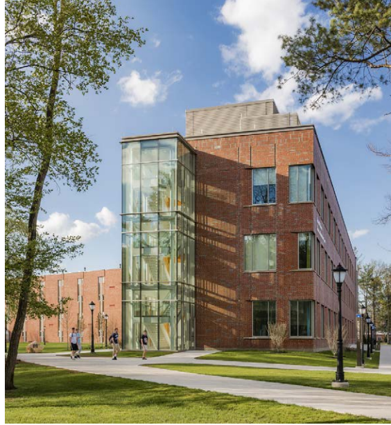
Glass-enclosed stair provides new landmark on Western Ave.
