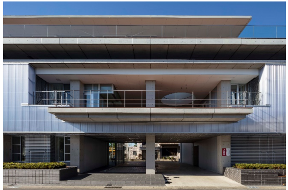
West-side view Approach
