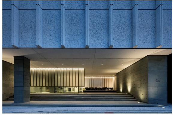
Entrance view from the North
