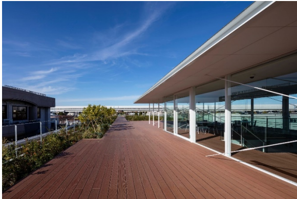
3F Roof terrace
