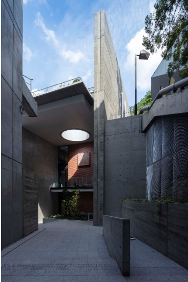
1F level approach
