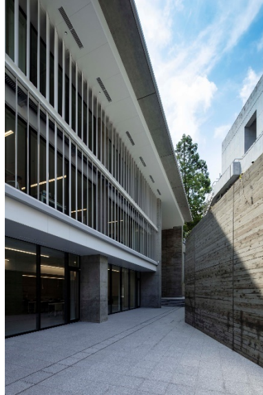
1F level approach
