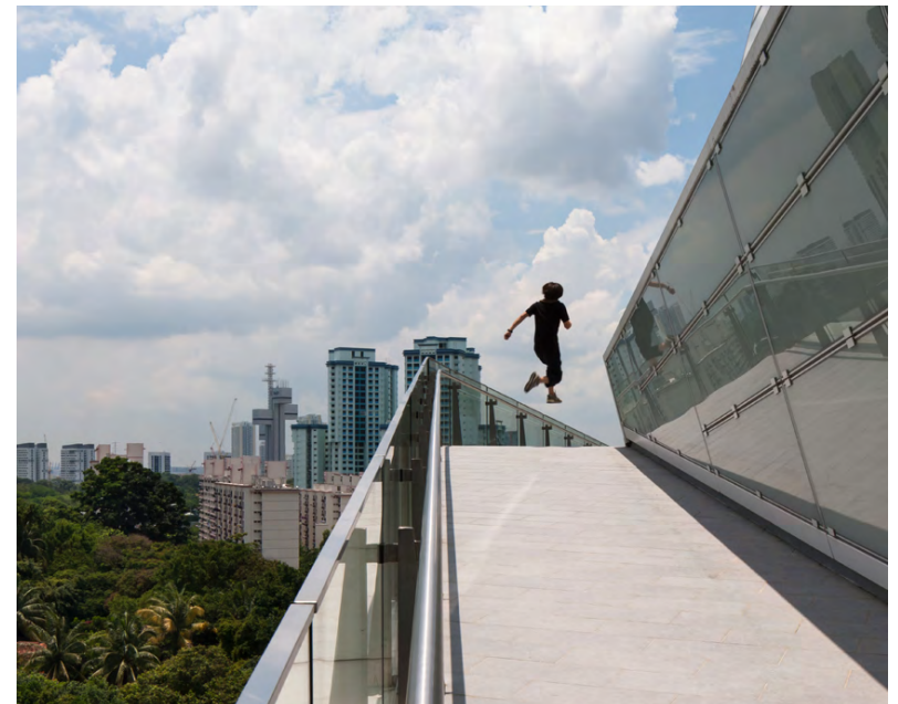
400m (1,300 ft.) public loop, 40m above ground
