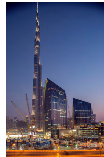
Northeast entrance, gateway to downtown
