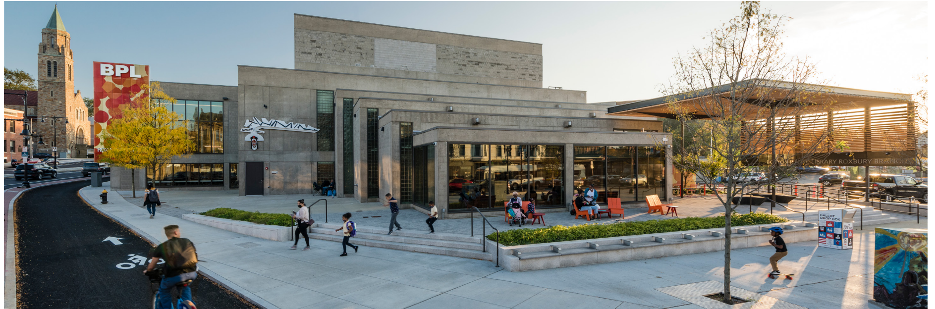
Roxbury Branch of the Boston Public Library Renovation, Roxbury, Massachusetts Credit: Anton Grassl Photography
