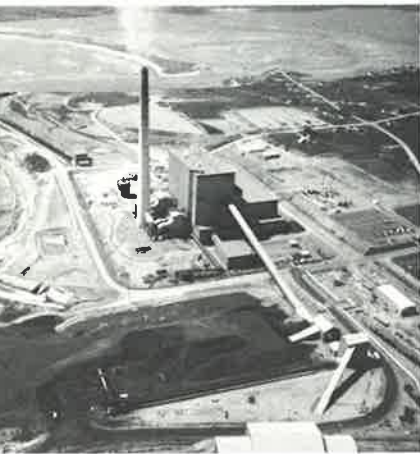
Lingan Power Generating Plant Lingan, Nova Scotia
