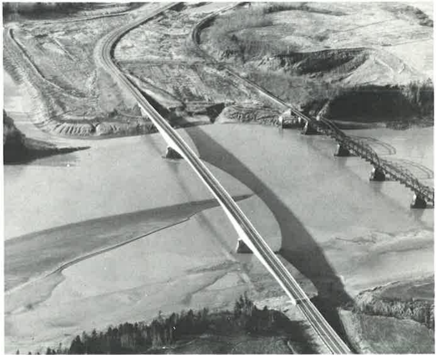
Clarence L. Gosse Bridge Shubenacadie River, Nova Scotia Honourable Mention Canadian Consulting Engineering Design Awards
