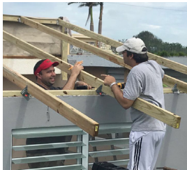
Helping rebuild Roofs after Hurricane Maria. Puerto Rico, 2017
