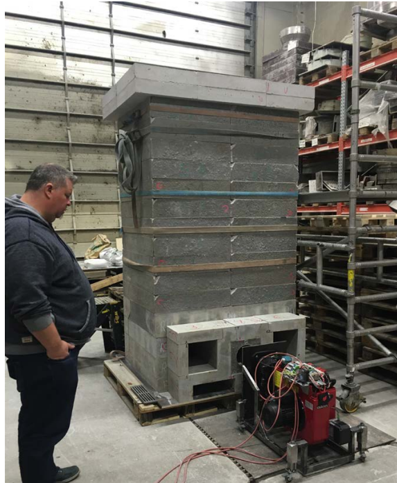
in-process construction photograph: custom stove from Finland
