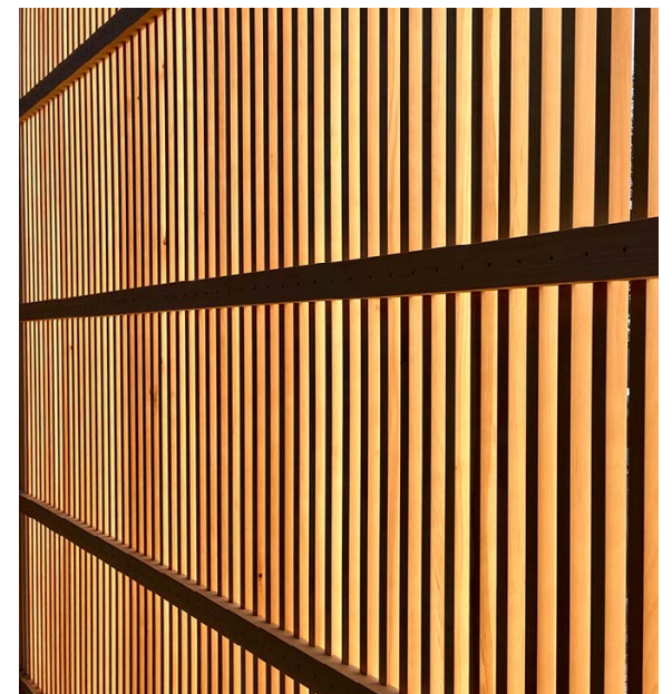
in-process construction photograph
