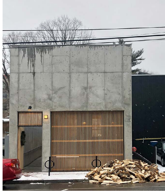
in-process construction photograph
