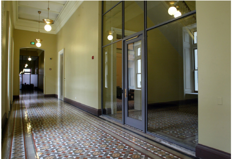
second floor corridor after
