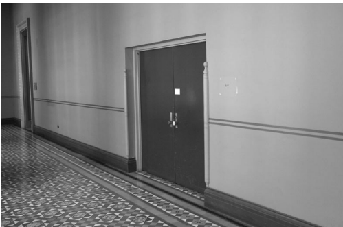
second floor corridor before
