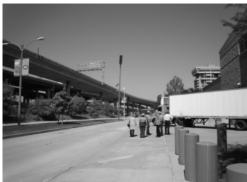
ranger station site before construction
