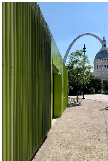
kiener visitor services building
