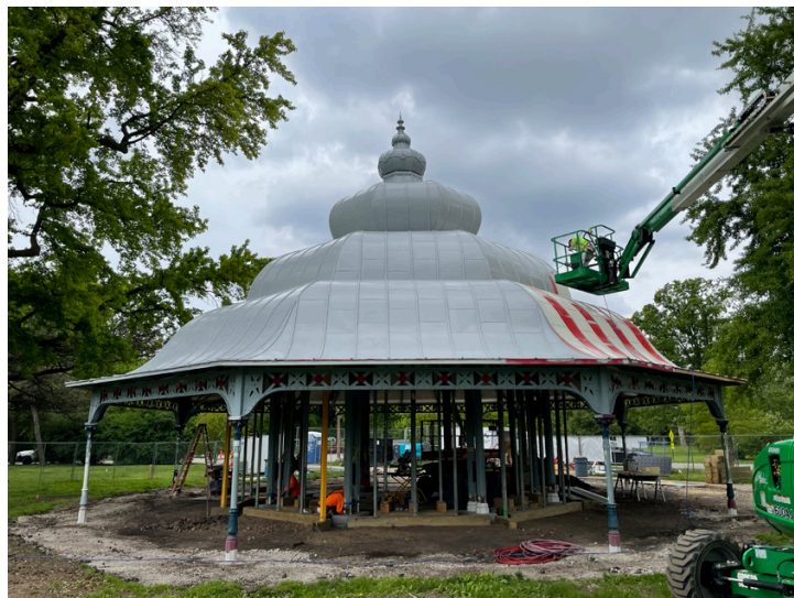
turkish pavilion during restoration
