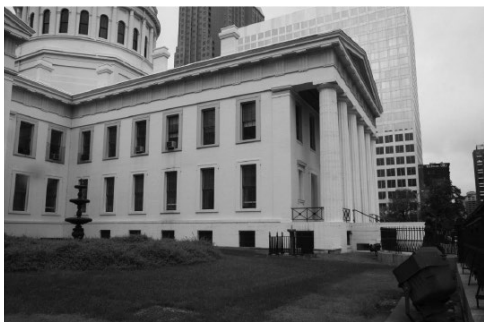
southeast courtyard before
