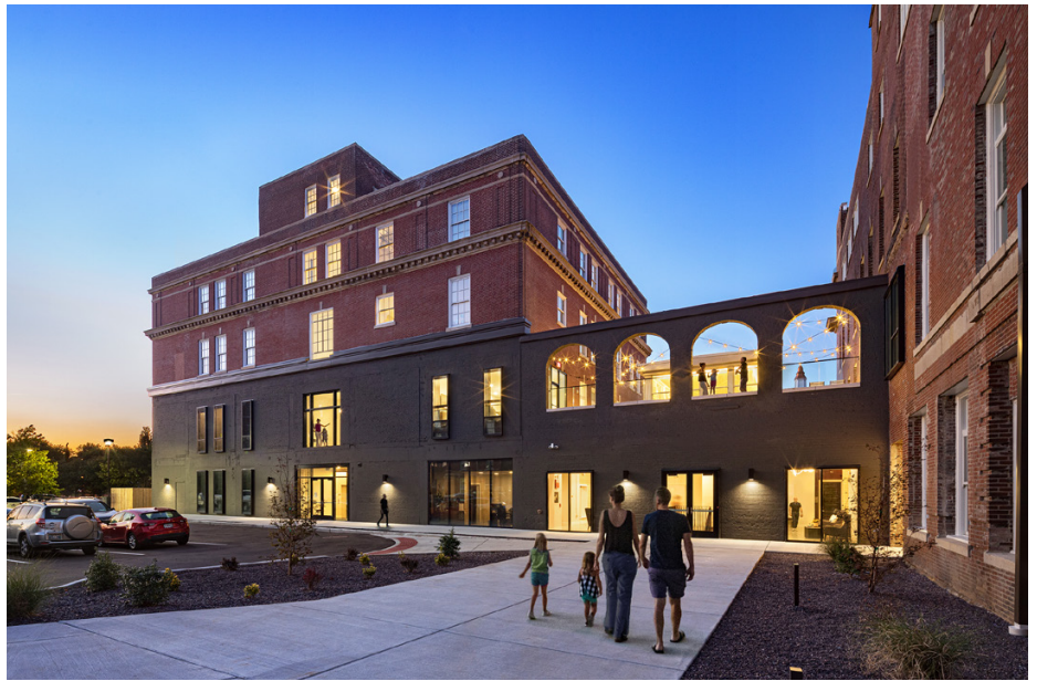
service building south exterior after
