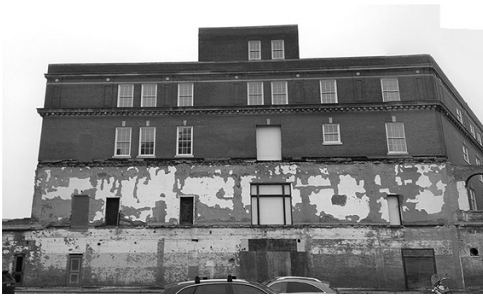
service building south exterior before
