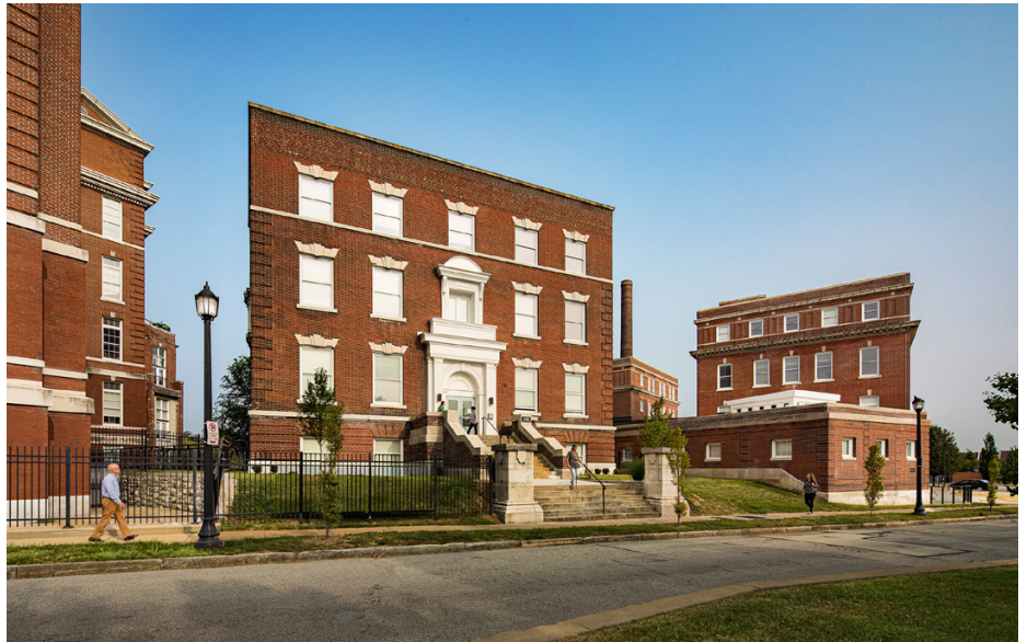
commissioner building east exterior after
