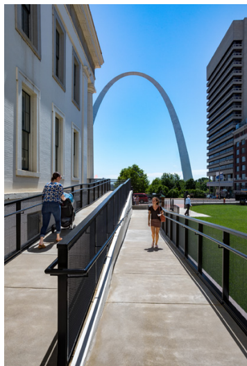
southeast courtyard ramps
