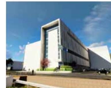
LOCKHEED MARTIN GATEWAY BUILDING Littleton, Colorado
