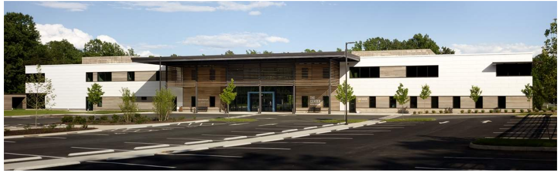
The Center at Belvedere, Charlottesville, VA, Bushman Dreyfus, Architects, AOR Douglas Gallow, Senior Center Design Specialist
