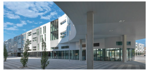
Plaza and first-floor retail space
