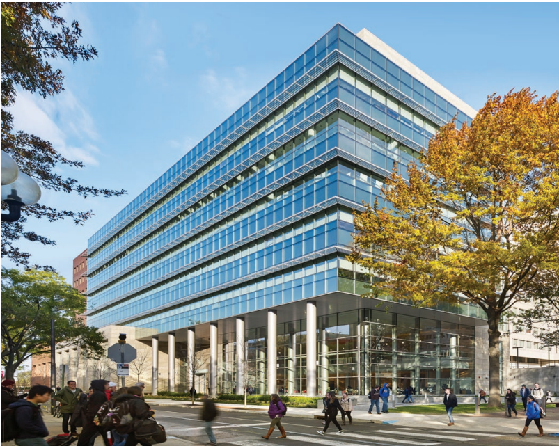
View toward main lobby on pedestrian thru-way, Polett Walk
