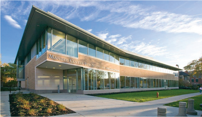
Main entrance along Bellflower Road
