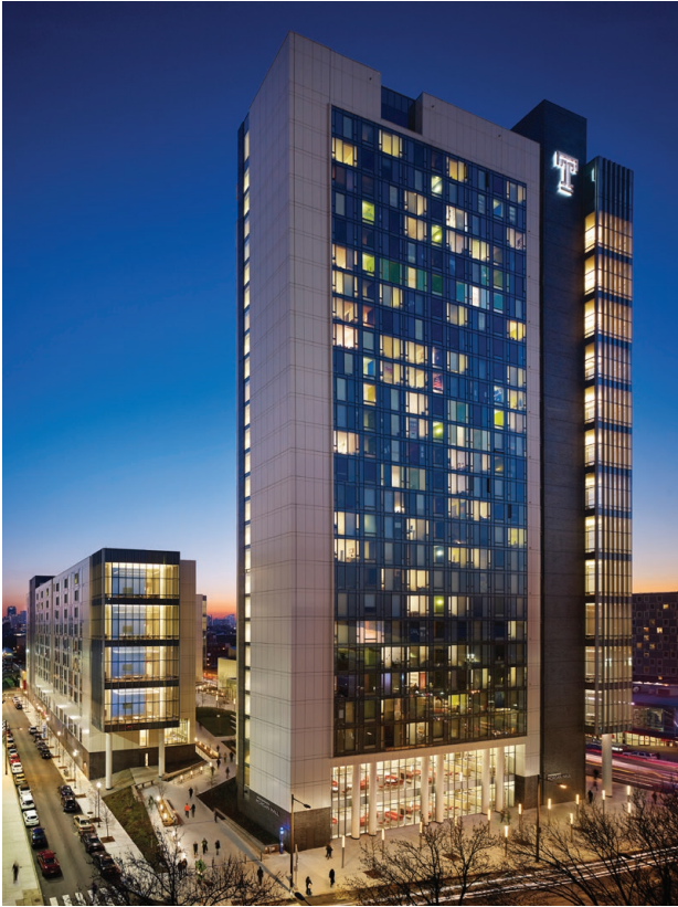
View of residential tower from campus
