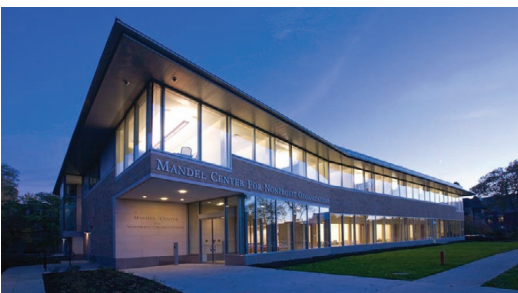
Main entrance at dusk
