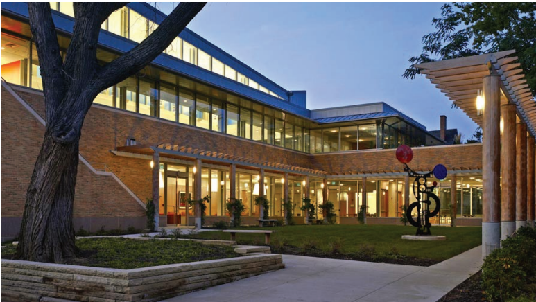
Garden surrounded by pergola; rooftop garden beyond
