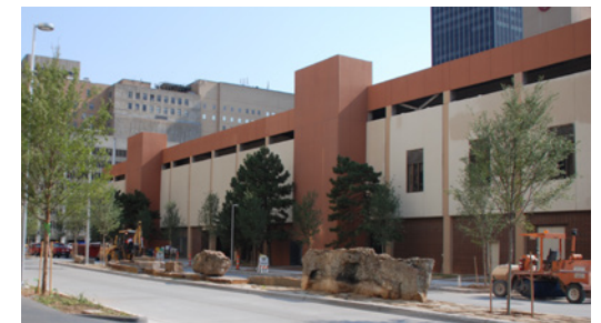
West facade of the building prior to construction.
