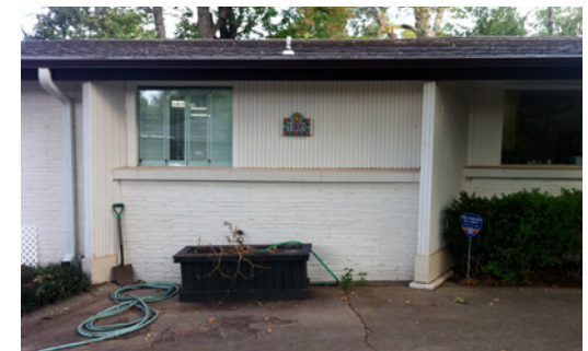
Woodland facade prior to construction.
