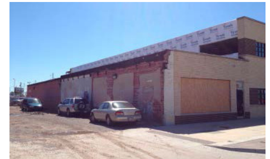
Abandoned building prior to construction.
