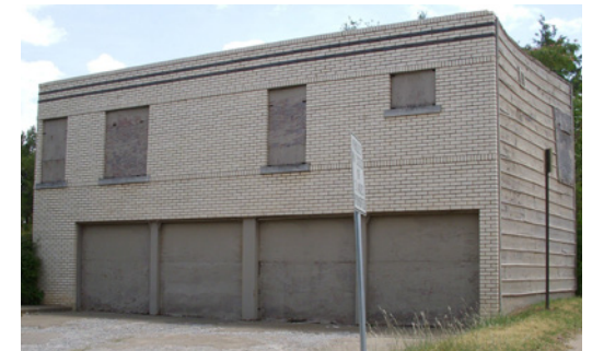
Garage prior to reconstruction.
