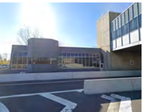
Goethals Bridge Operations Center Building Project Architect Staten Island NY—Elizabeth, NJ
