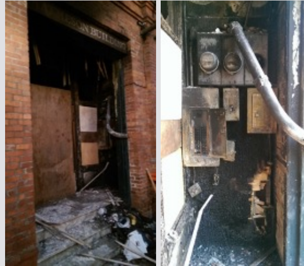
Electrical panel post-fire
