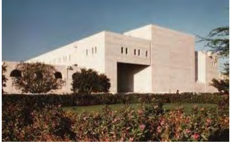
View from the Roadway Above
