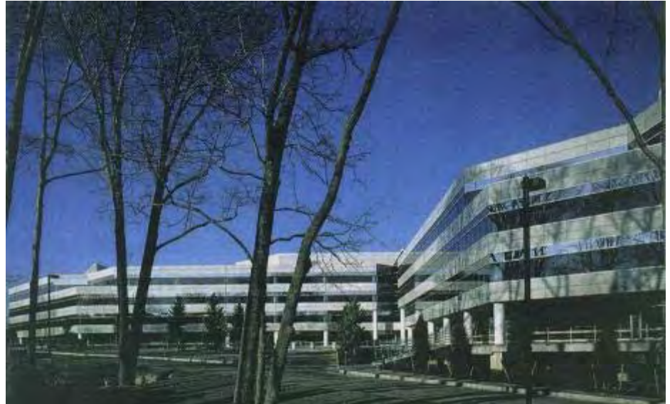
View Towards 100 Summit Lake Office Entry Above
