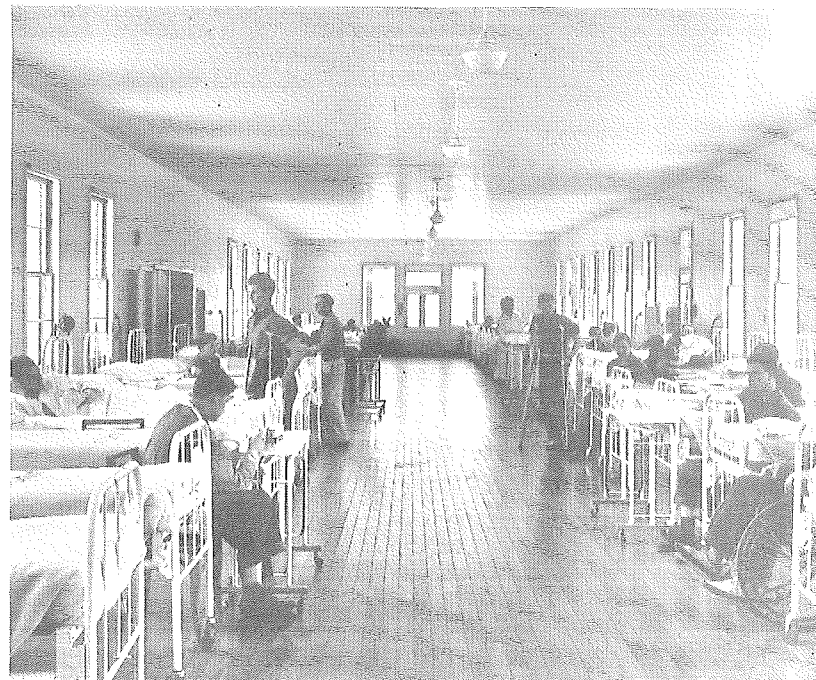
WARD INTERIORS ARE SOUND ABSORBING PLASTER BOARD
