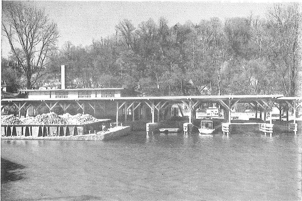
GRAVEL SPREAD ON THE RIVER BOTTOM PREVENTS EROSION NEAR DOCK
