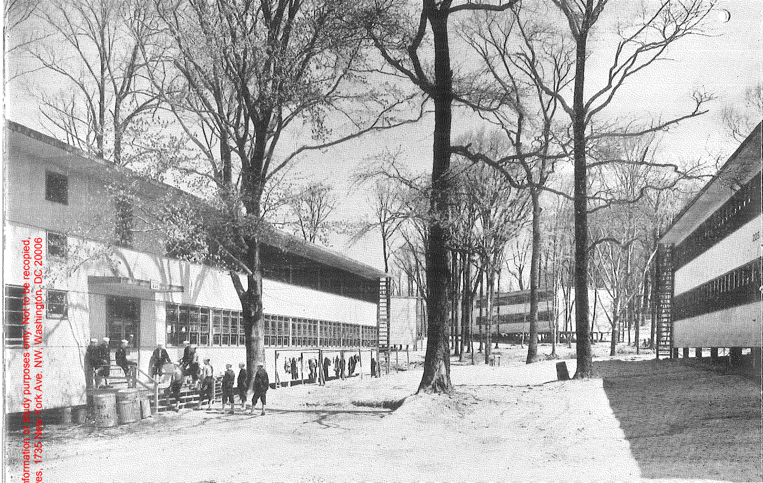
GENEROUS SPACING OF BUILDINGS SAVED MANY LARGE TREES. OVERHANGS PROTECT THE TEMPORARY EXTERIORS
