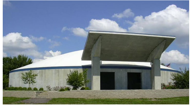
The unique shape of the shelter's curved surfaces force the wind around the shelter on all sides
