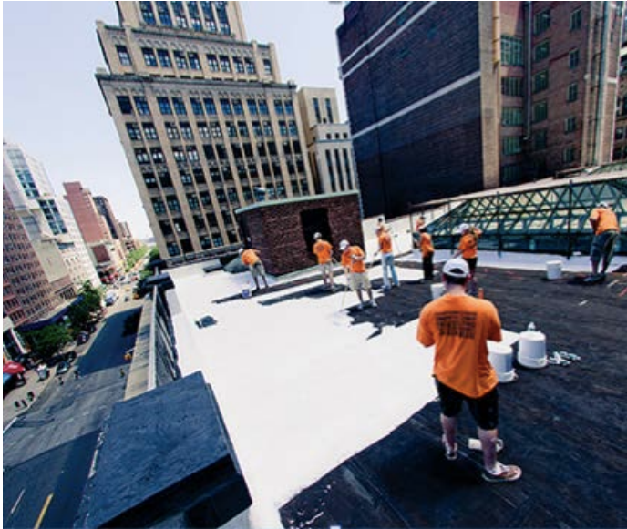
Princeton University students painting a roof white in New York City.
