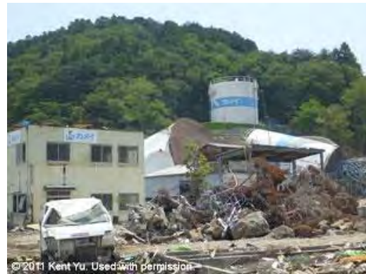
Figure 16-6: Steel tanks damaged due to Tohoku, Japan Tsunami in 2011
