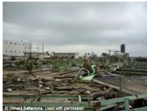
Figure 16-14: Sendai WWTP equipment and piping damage from the 2011 earthquake
