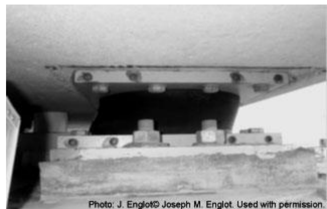
Figure 13-11: Airtrain seismic isolation bearing
