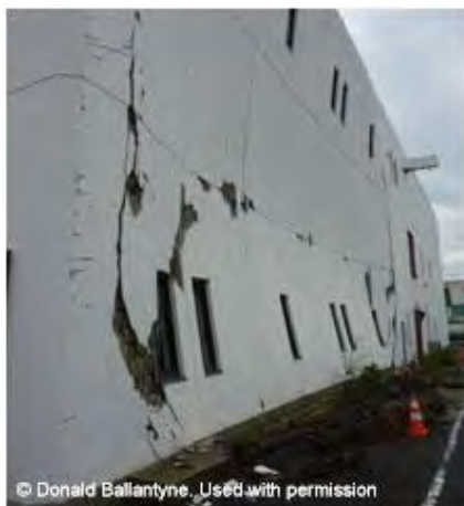
Figure 16-13: Sendai WWTP Effluent Pump Station damaged by Tsunami in 2011 Tohoku Earthquake
