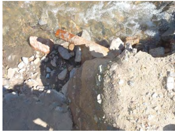
Figure 16-9: Exposed (left) and broken(right) distribution lines resulting from flooding in Jamestown, CO [Source: Environmental Protection Agency]
