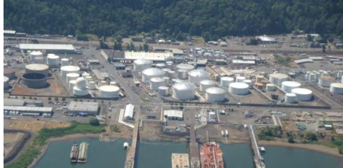
Figure 11-7: Portland, OR liquid fuel tank farm is vulnerable to failures in pipelines in Washington State. (Source: Yumei Wang [DOGAMI 2012])
