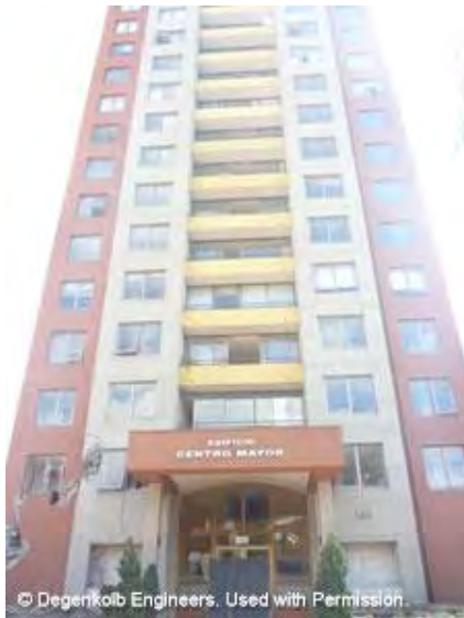
Figure 12-8: Apartment building with damaged structural members that is structurally stable
