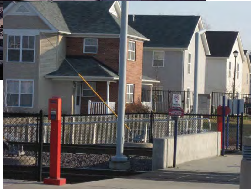
Emerson Park MetroLink Station East St. Louis, IL
