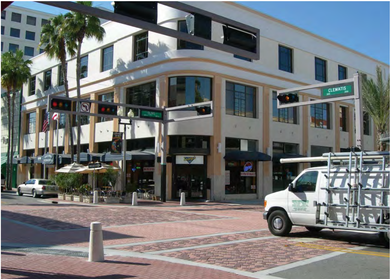
Facing problems with speeding, cut-through traffic, and safety, the City of West Palm Beach worked with concerned neighborhoods to develop traffic-calming solutions, including paved intersections, landscaping, bollards, curb bump-outs, and improved signage. Photo: Carissa Schively.
