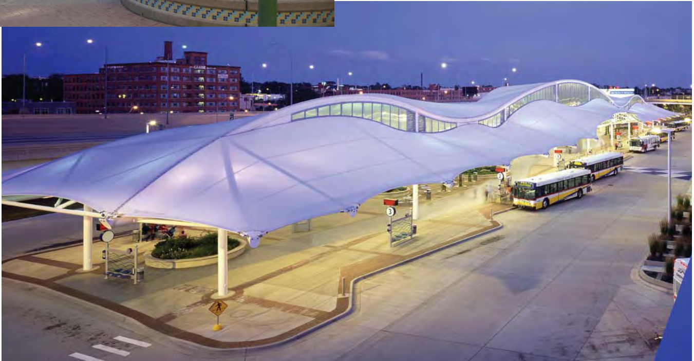
Bottom: The Rapid Central Station in Grand Rapids, Michigan, is located on a reclaimed brownfield; it features a green roof that reduces stormwater runoff and maintains temperatures in the building. This project used LEED guidelines and was the first LEED-certified transit facility in the country. Photo: Chuck Heiney Photography. Courtesy Progressive AE.
