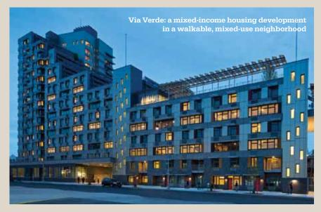
exposure, stepping the massing of the building down from a 20-story tower at the north to a mid-rise building, which in turn steps down from 13 to six stories; four- and twostory townhouses make the next steps, and finally an amphitheater steps down to a central courtyard at ground level.
