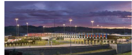
Mariposa Land Port of Entry Jones Studio (Architecture) Timmerman Photography
