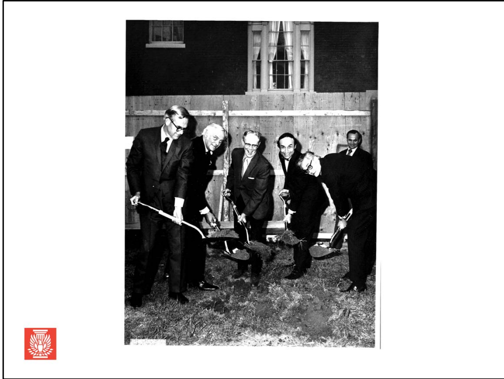
Groundbreaking for the new building happened on April 22, 1971.
