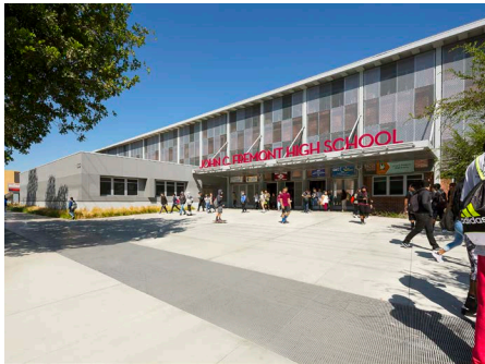
Fremont High School Modernization Los Angeles, CA
