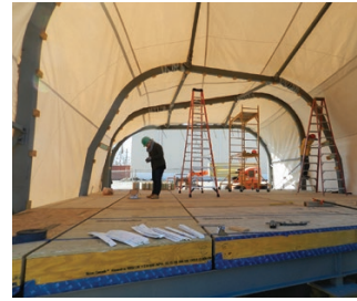
Figure 6. Taping of the floor pallets.
