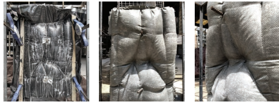
▲ Figure 10. System-B control cast; photo series of the control cast, further investigating the location tolerances of the mechanical anchors and the secondary weaves' ability to respond to varying lateral pressure in the formwork.
