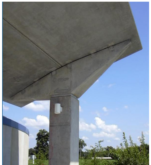
Canopies mounted on concrete piers designed to withstand 250-mph winds provide weather protection
