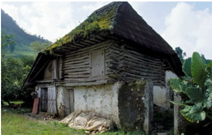
Hidalgo, Mx. Log cabin supported by masonry ground level structure, wood shake roof
