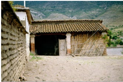
Oaxaca, Mx. Ceramic "hat" protecting adobe wall
