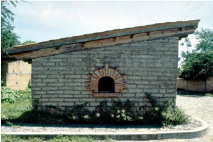
Puebla, Mx. brick window frame in shed roofed adobe
