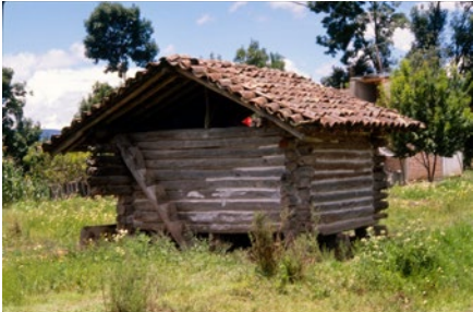
Morelos, Mx.- “Troje”- grain silo: hand hewn logs on stone piers with wood fired clay tile roof
