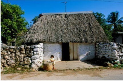
Yucatan, Mx. Casa Maya, lime stucco over wattle and daub walls, thatch roof
