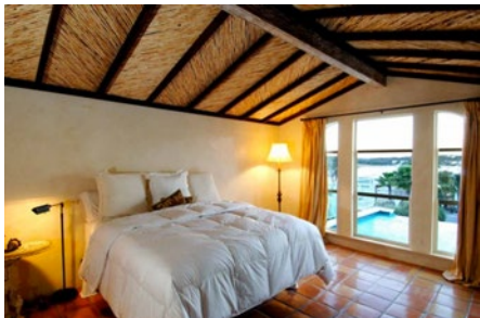
Lakeway, Tx.- "Latilla" ceiling at master bedroom of Ballas remodel
