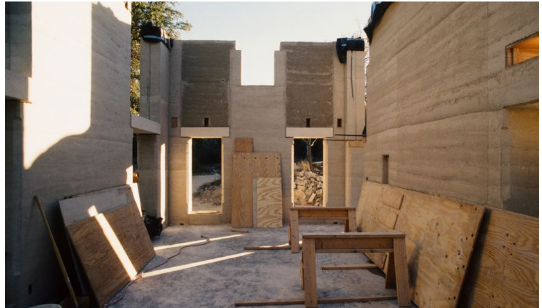
top left: chamfered edge niche in "caliche" rammed earth wall top right: Double height living area with heavy timber truss gable roof on rammed earth load bearing walls. above: Under construction, double height interior space created by load bearing, rammed earth walls
