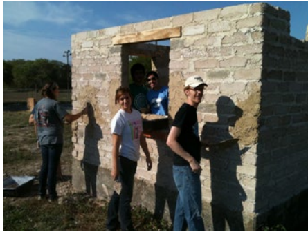
Texas A&M students building compressed earth block (CEB) structure
