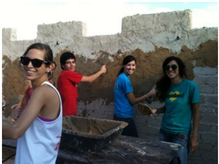
Texas A&M students applying adobe stucco on CEB structure
