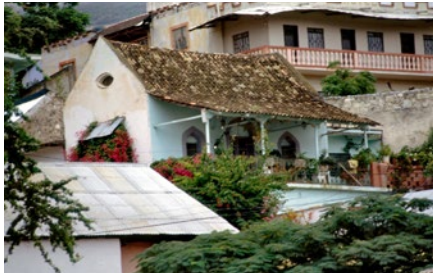
Veracruz, Mx. Ceramic wood fired clay roof for gable and porch
