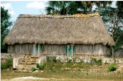
Yucatán, Mx. Casa Maya, absidal shape dwelling. Reed walls on stone base; thatch roof
