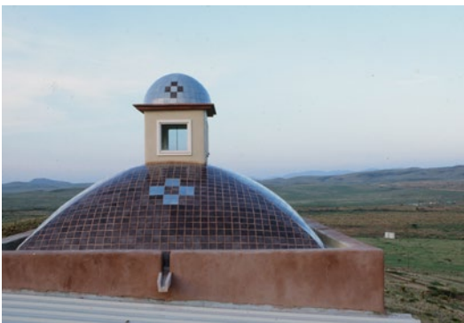
upper left: General view of Las Auras adobe residence upper right: Bovedero (dome builder) Alfredo Avila setting the "spring" for the next boveda (dome or vault). Note the daylight gathering lantern of the previous boveda in the background. lower left: Finished boveda clad with ceramic tile lower middle: Gaggles of auras (buzzards) painted by artist Mahala Sibley lower right: Under construction boveda sin cimbra (centerless vault)
