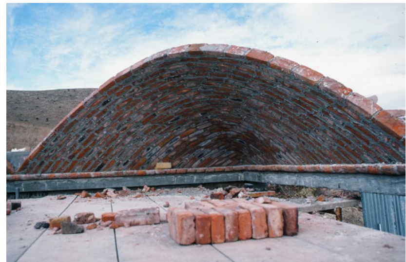
upper left: General view of Las Auras adobe residence upper right: Bovedero (dome builder) Alfredo Avila setting the "spring" for the next boveda (dome or vault). Note the daylight gathering lantern of the previous boveda in the background. lower left: Finished boveda clad with ceramic tile lower middle: Gaggles of auras (buzzards) painted by artist Mahala Sibley lower right: Under construction boveda sin cimbra (centerless vault)
