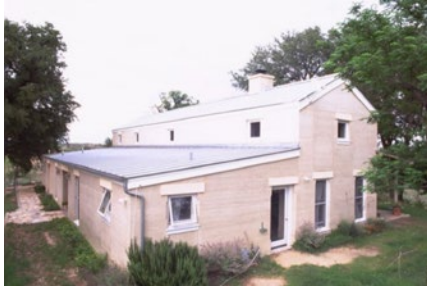
Knikerbocher, Tx.- Spring house- “caliche”rammed earth dwelling
