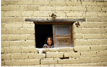
Michoacan, Mx. A smile through the window with a mesquite lintel of an adobe dwelling
