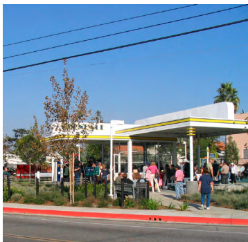
ADAMS SQUARE MINI-PARK, Glendale, CA City of Glendale Completed 2007
