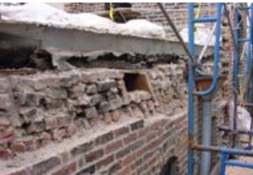
(BEFORE) Portion of wall removed to inspect masonry deterioration
