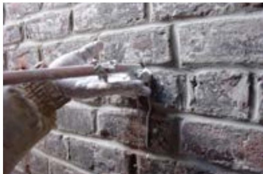
(PROCESS) Mortar injection installation
