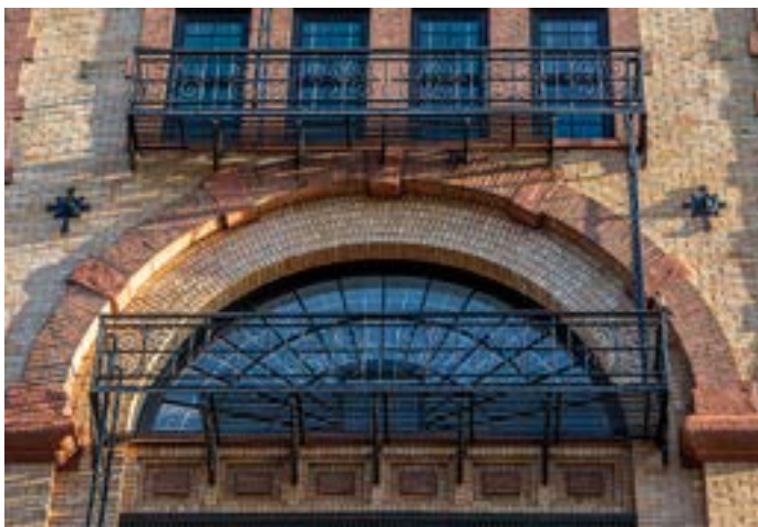
(BEFORE) Image from 1978 designation report (AFTER) Cast iron balcony restoration and masonry reconstruction
