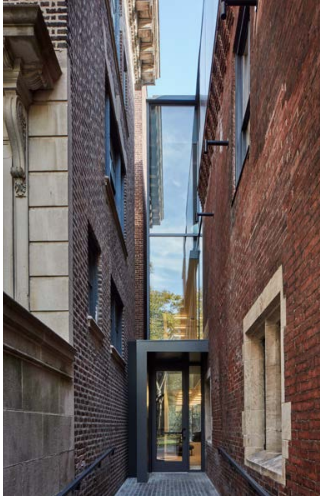
(AFTER) Integration of modern addition with historic building fabric
