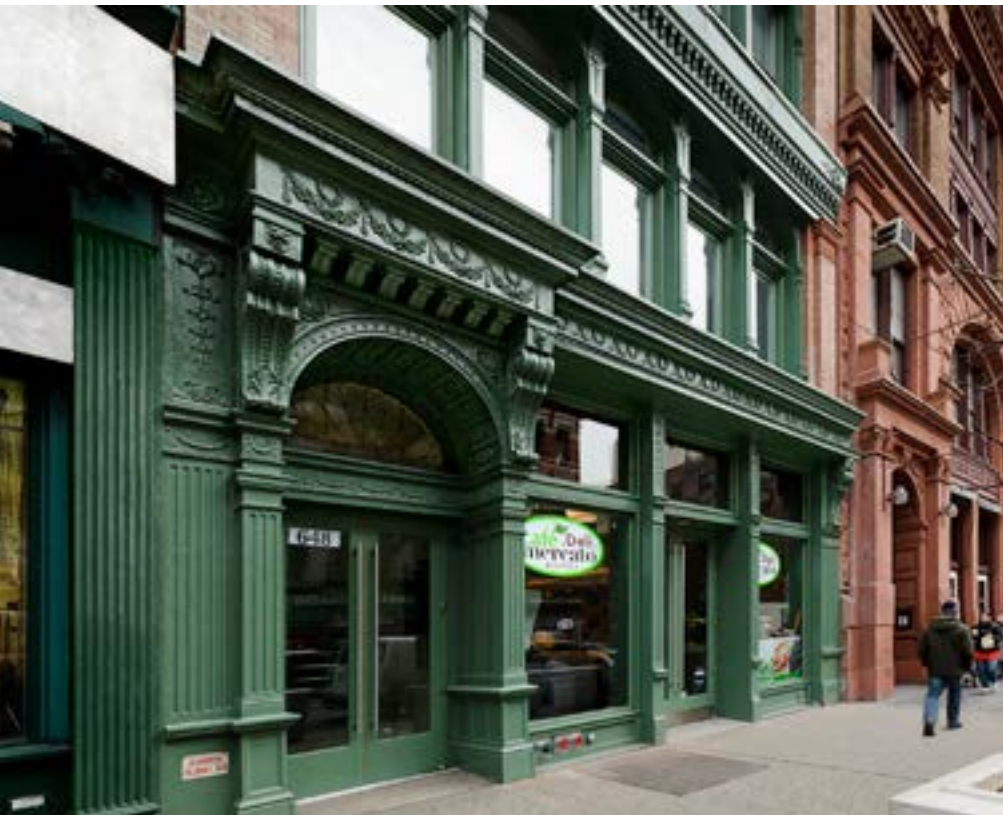
(AFTER) Restored Victorian cast-iron storefront facade after removal of 20th century accretion
