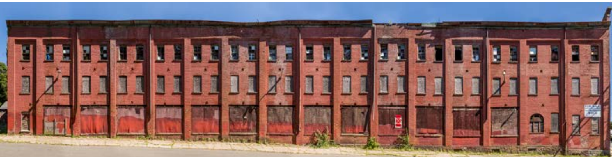
(BEFORE) Exterior prior to restoration
