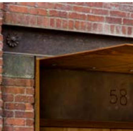
(AFTER) Exterior detail of doorframe
