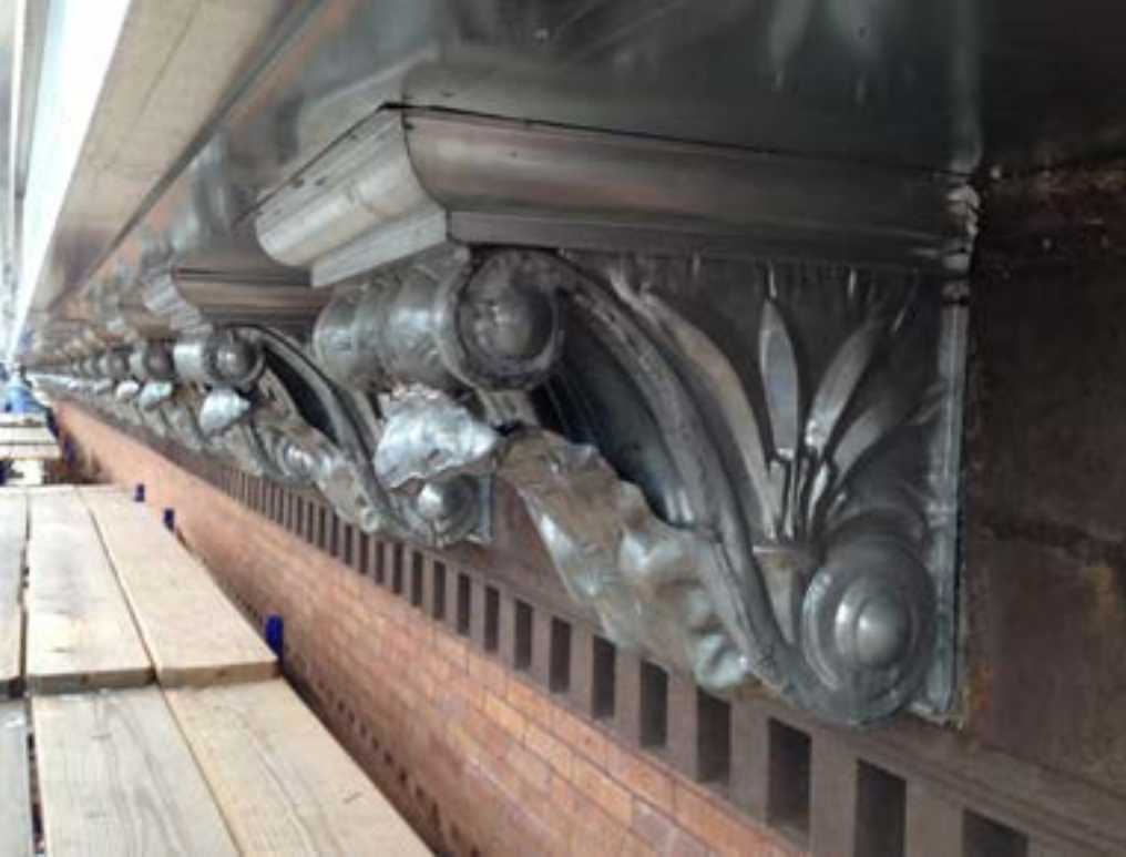
(BEFORE) Exterior exposed cornice prior to restoration
