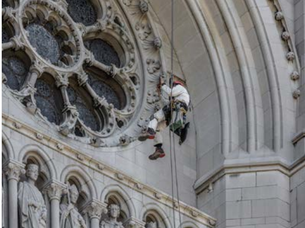
Worker performing visual exterior inspection depicted above
