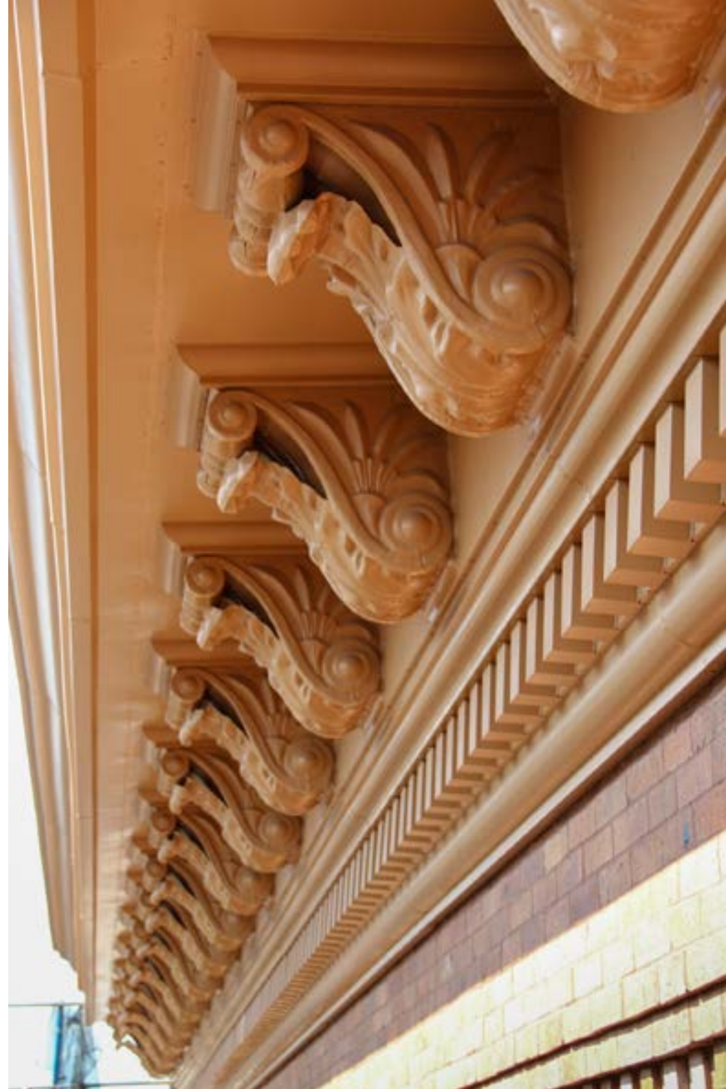
(AFTER) Restored pressed tin cornice detail
