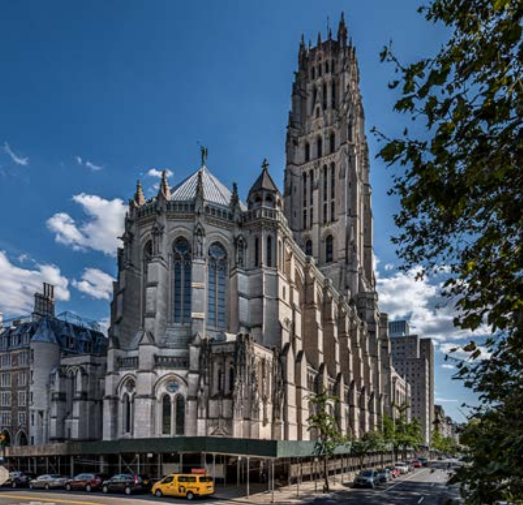
Steel frame construction of the church allowed for the lofty height of the tower
