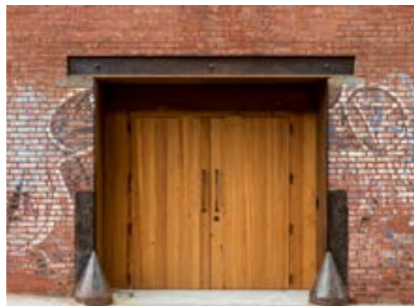
(AFTER) Detail of doorway with cast iron lintel
