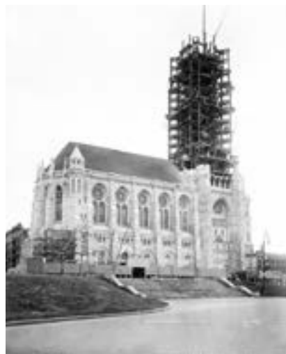
Steel frame of tower clad with limestone, c. 1930
