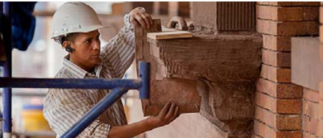
(PROCESS) Worker running mold for window sill trim
