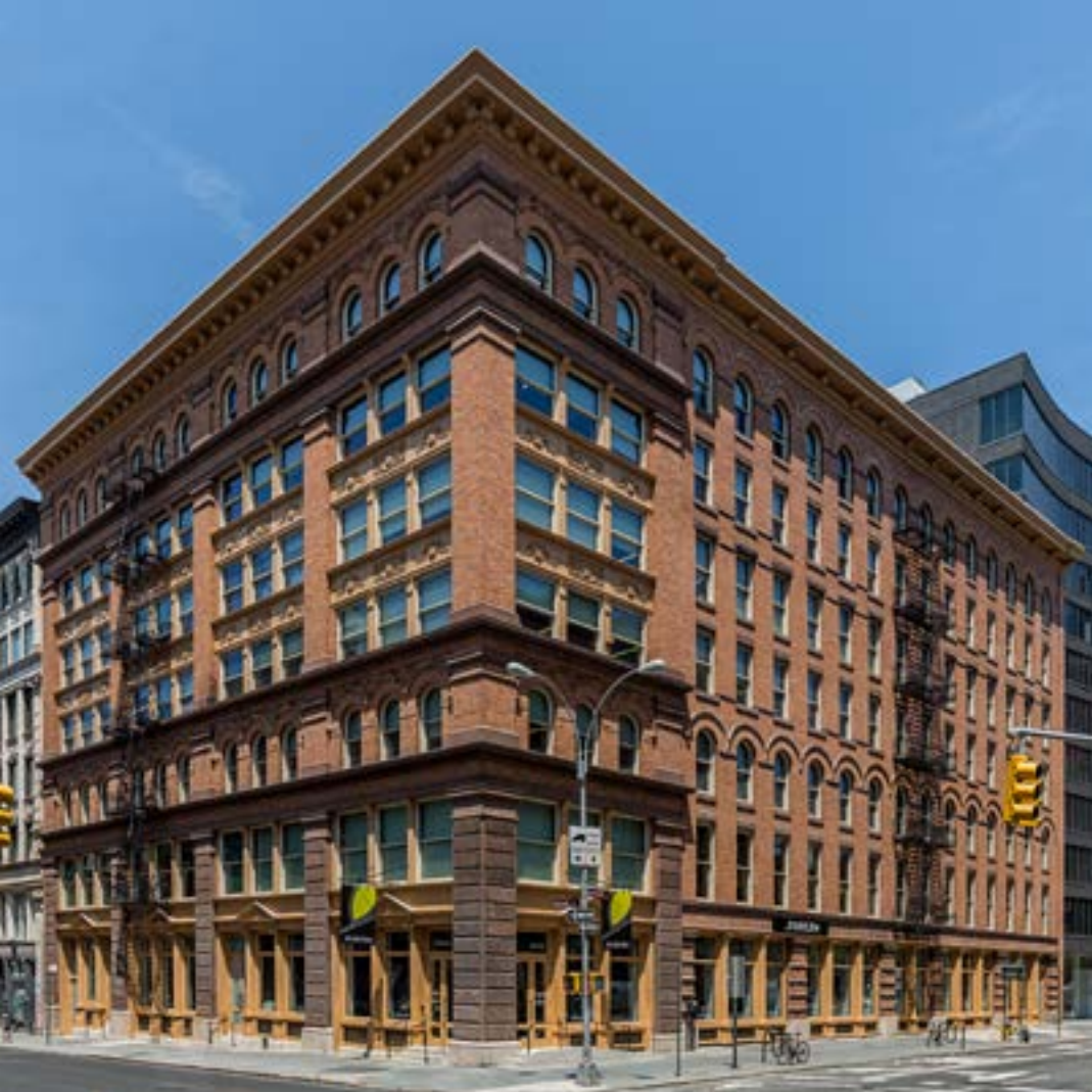
(AFTER) Knickerbocker Building following restoration of deteriorated brownstone and cast iron elements
