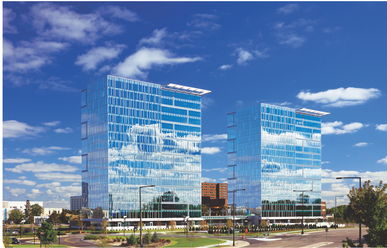
Residential Towers with Floor to Ceiling Glass Open Up Views to the Wildlife Refuge & River
