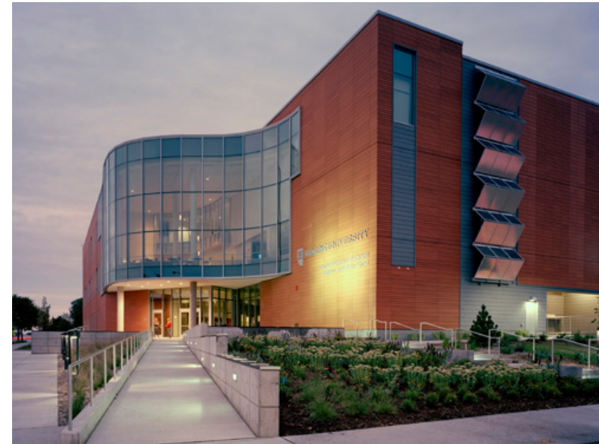
Public Street Entrance
