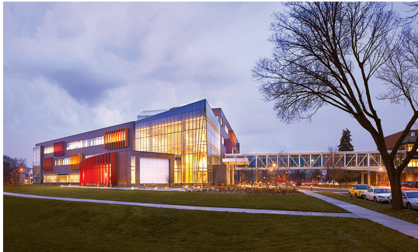
Exterior facade from campus mall
