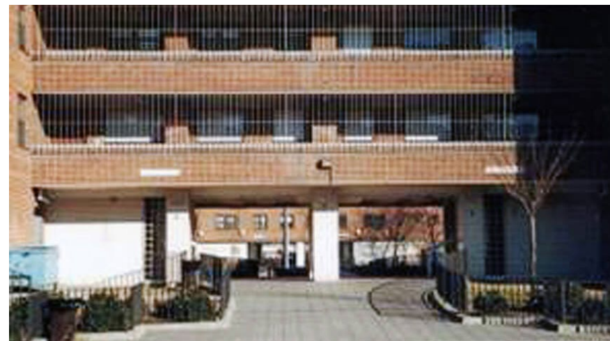
View of Bayside Lobbies. Left, after transformation by enclosure of breezeways, addition of new fire stairs, and connecting balconies with apartments. Right, before transformational changes, when open breezeways and “outdoor terraces,” part of the fire egress, both posed security problems for residents.
