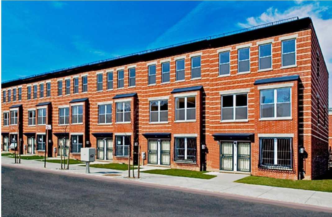
View of new, Two-Family Townhomes — this building type being an updated version of the Brooklyn rowhouse.
