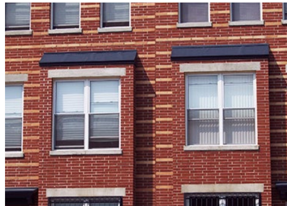
Detail, showing paired bay windows, brick pattering, and stone details.
