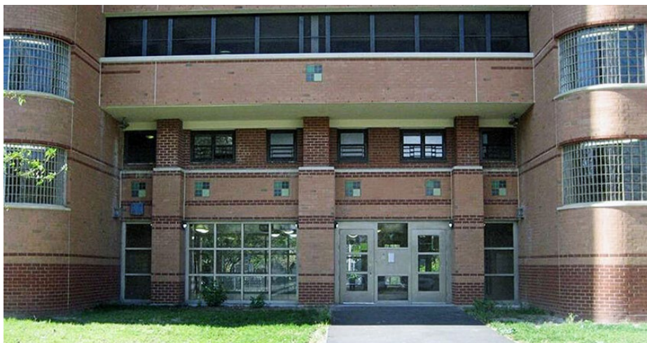
View of Bayside Lobbies. Left, after transformation by enclosure of breezeways, addition of new fire stairs, and connecting balconies with apartments. Right, before transformational changes, when open breezeways and “outdoor terraces,” part of the fire egress, both posed security problems for residents.
