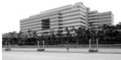
The existing building, prior to renovation, lacked proportion and grace.
