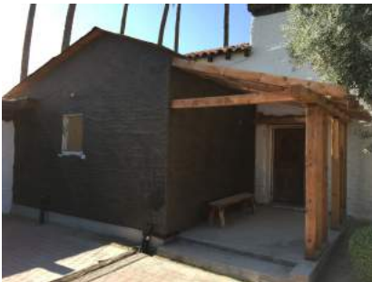
Addition under construction
