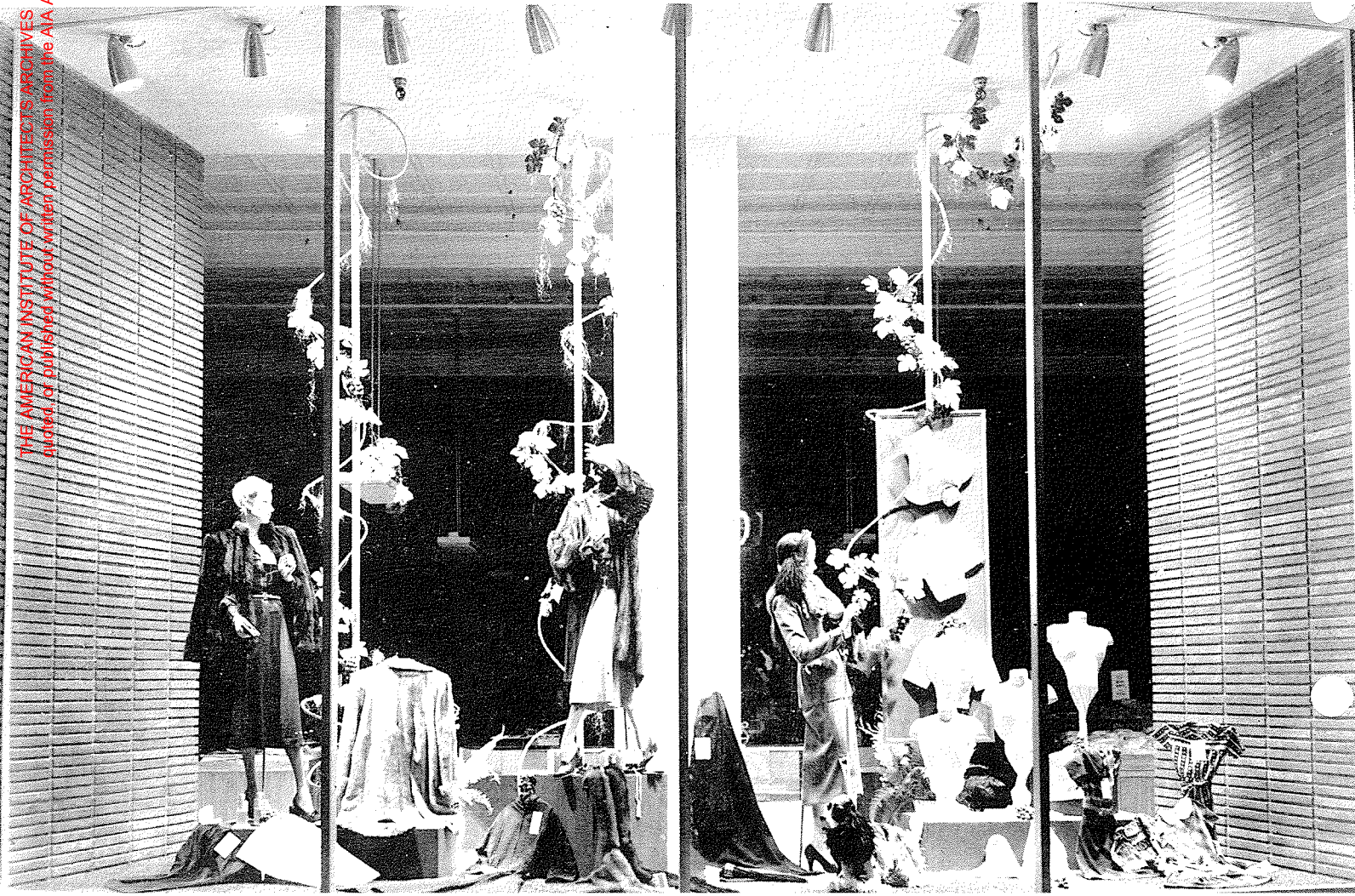
Detail of display window. Unadorned roman brickwork in stack bond offers modern setting for merchandise.
