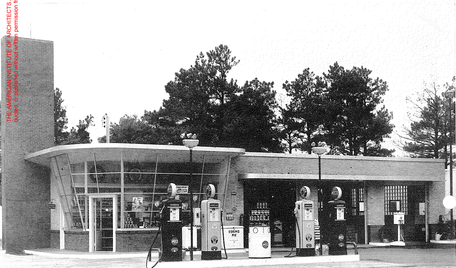
Travis Oil Company features red brick with red mortar and gray brick with natural mortar.
