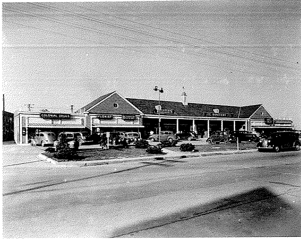
SHOPPING CENTER ARLINGTON VIRGINIA 9 STORES $ 85,000 FOR GARFIELD KASS
