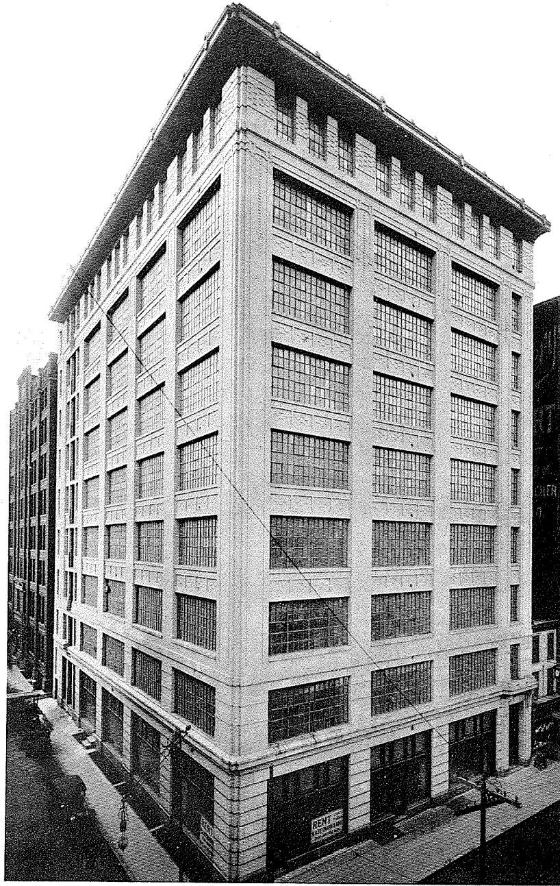
METZGER BUILDING, PHILADELPHIA
