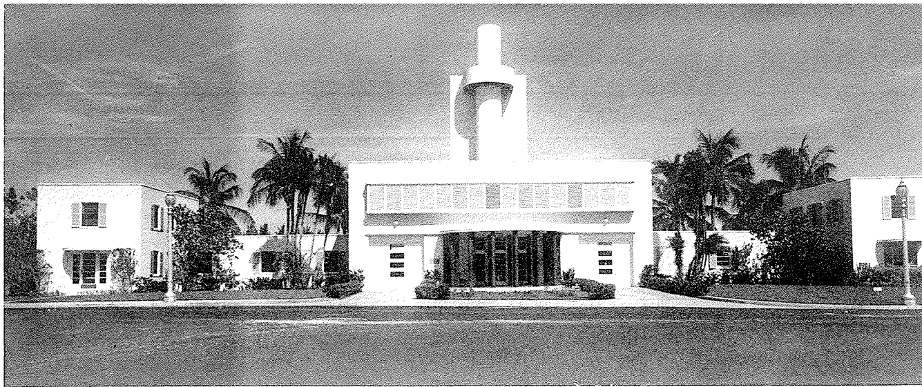
DADE BOULEVARD FIRE STATION, P.W.A. PROJECT MIAMI BEACH, FLORIDA
