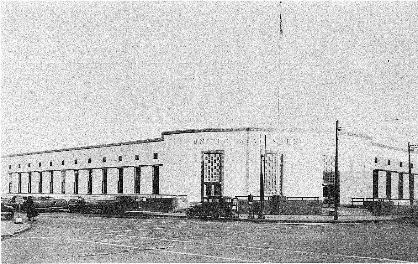
NEW ROCHELLE POST OFFICE
