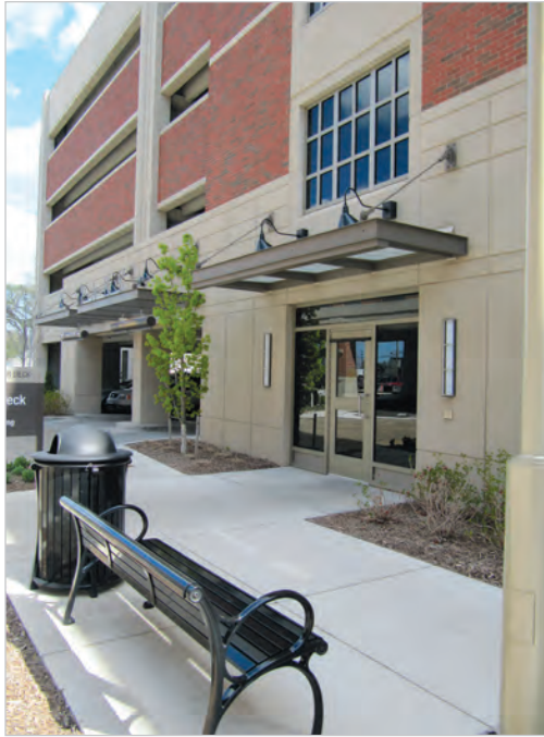
Figure 9: Parking structure entrance
