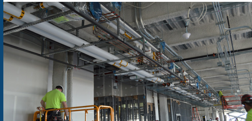
MEP racking systems installed
