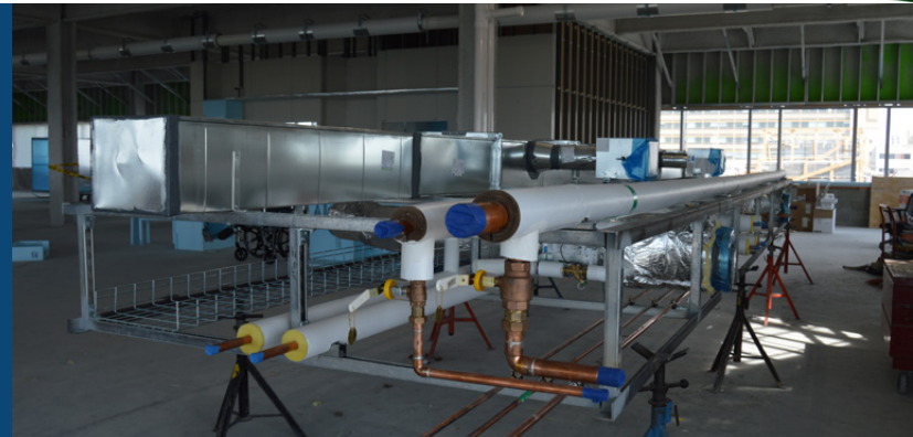
MEP racking systems prefabricated in the shop
