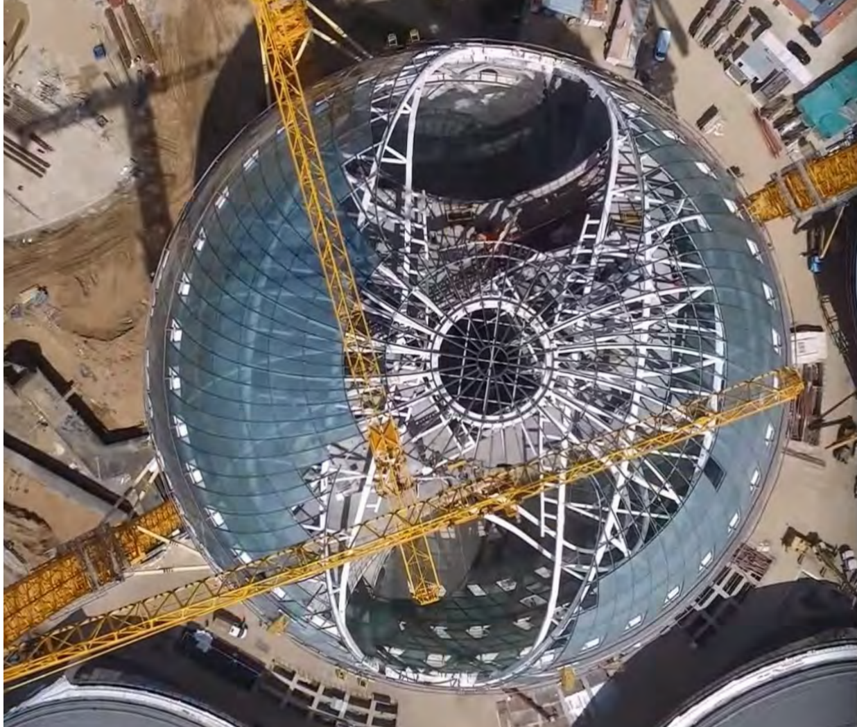
Kazakhstan Pavilion Construction Photograph
