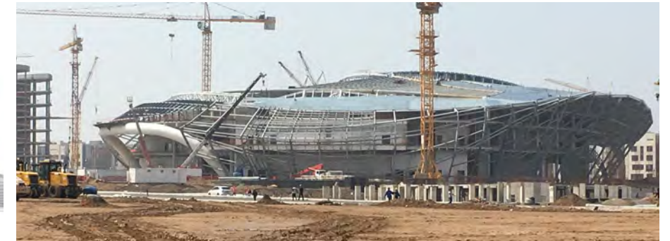
Congress Center Construction 2016
