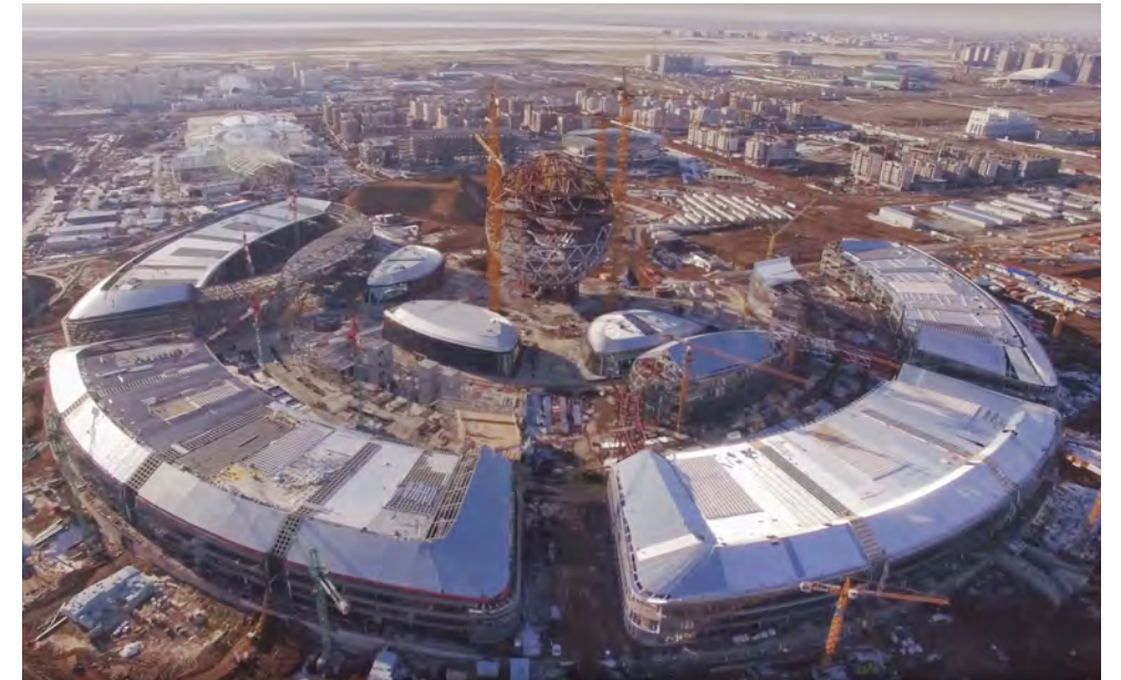
Construction Site June 2016
