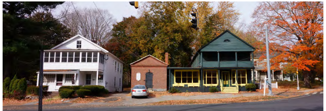
Empty commercial buildings along Woodbury's Main Street.
