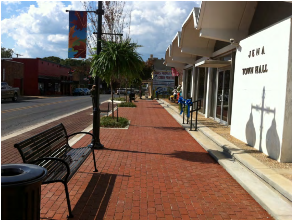
Town of Jena's improved streetscape completed in collaboration with LaDOT.
