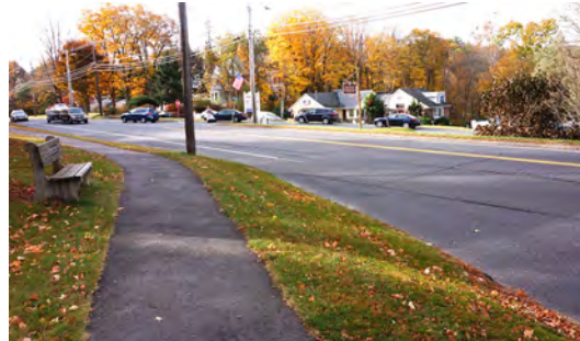
Typical asphalt on grade sidewalk.
