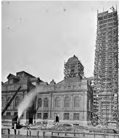
Baltimore, MD sewage lift station.
