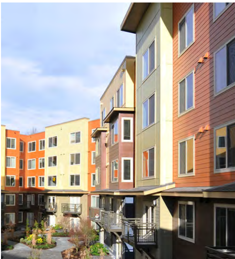
Multi-level senior care residence.
