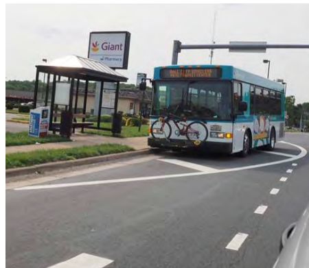
Existing far-side bus stop with sidewalk access is easier to access and does not conflict with right turns or through traffic.
