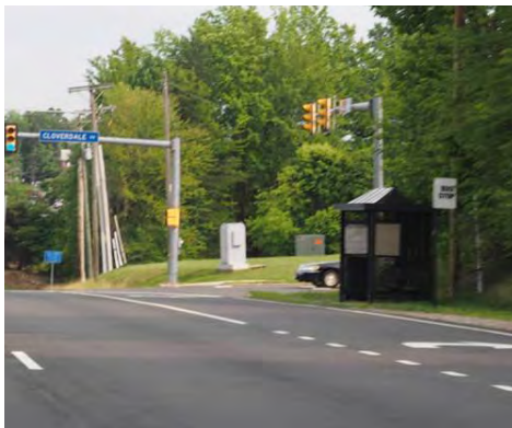
Existing near-side bus stop without sidewalk access is difficult to access and conflicts with right turns.
